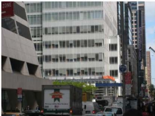
Photographs. One Bryant Park Progress Photos, 12 May 2009.
